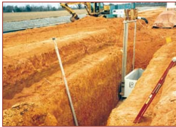
An active Slit Trench with disposal vault in place.
