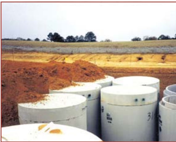
Cylindrical B/C Trench disposal vaults in an active trench. Vaults are immediately backfilled to fill void spaces and reduce radiation exposure.
