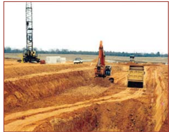
A typical B/C Trench under construction.
