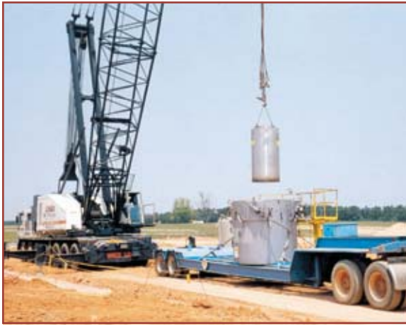
Transport Vehicle in position for removal of LLRW container prior to disposal in a B/C Trench.
